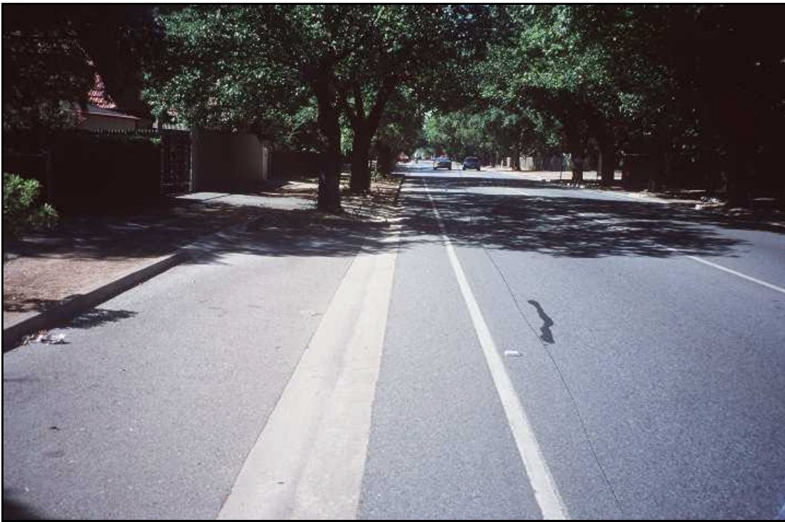
Figure 4: Arterial Road 4 with Parking Bays and Cycle Lanes
