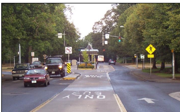
Figure 13: Two-way central bus lane splits at a bus stop, Eugene OR, US
