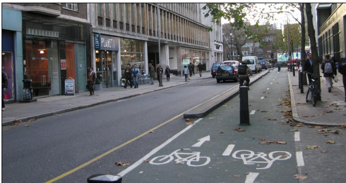
Figure 4: Removal of two-way traffic in London to allow for a separated cycleway
