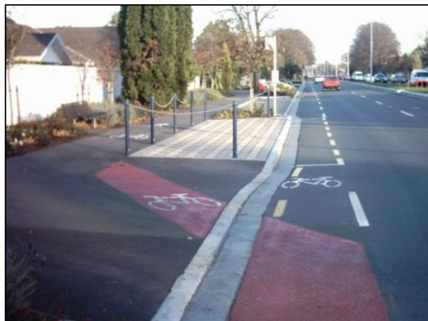
Figure 10: In-lane bus stop, Fendalton Rd, Christchurch, with bike bypass
