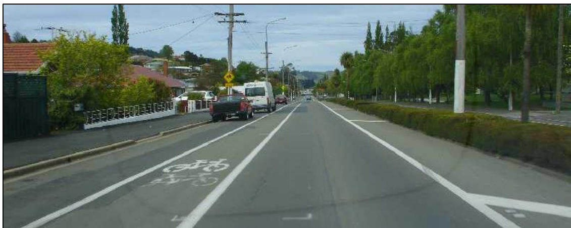
Figure 2: Road diet conversion from two traffic lanes, Kaikorai Valley Rd, Dunedin
