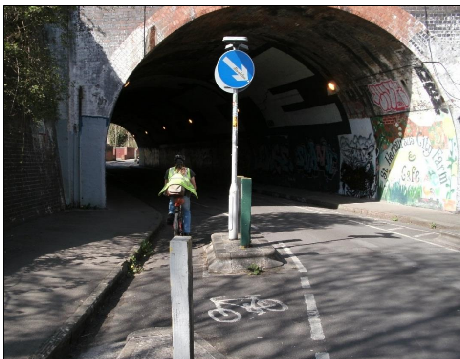
Figure 20: Cycle lanes either side of a single traffic lane, Mina Rd tunnel, Bristol UK
