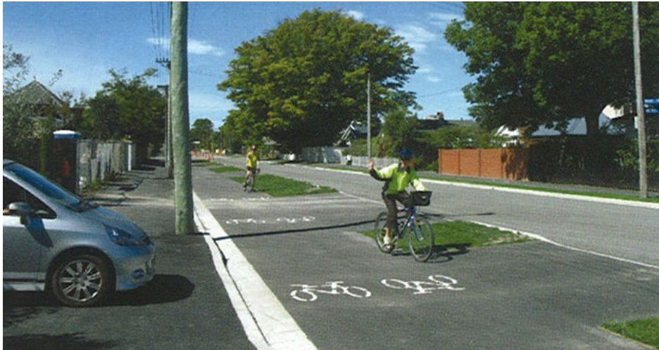
Figure 21: Matai Street West off-road cycle path
