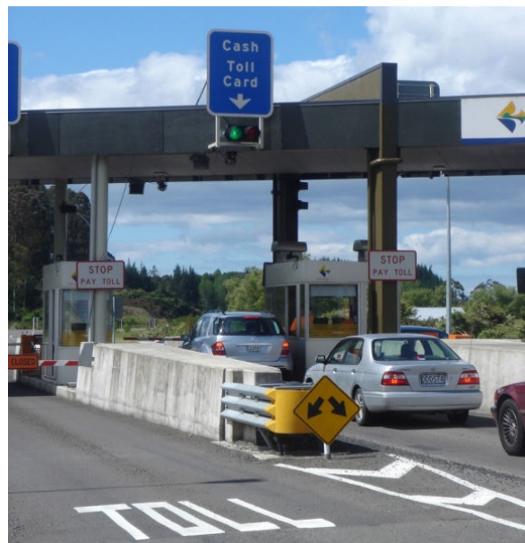
Figure 25: Tauranga’s Route K toll booth
