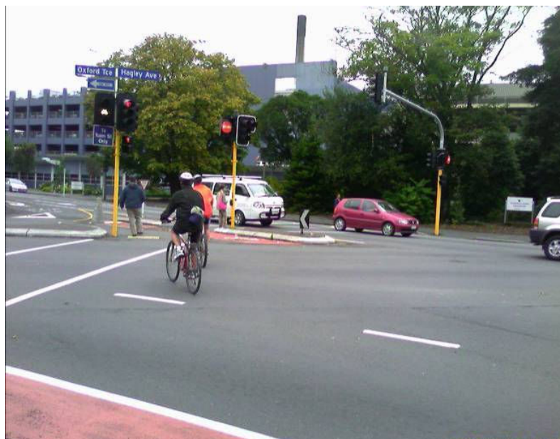
Figure 19: Cyclists cross the Oxford Tce/Riccarton Av intersection at protected signal crossing to access contra-flow cycle lane on Tuam Street
